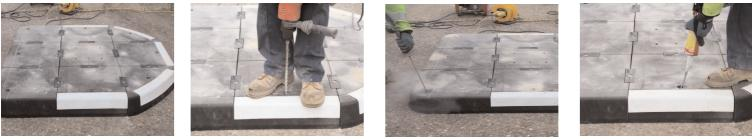
**6.** Repeat drilling, blowing, resin for remaining middle holes and use the black plastic anchor fixings to secure island. Once middle sections have been completed, drill remaining outside holes and blow out fixings holes using the long nosed air gun. Thoroughly blow out holes and insert resin commencing at base of hole, 2 to 3 pumps required.
