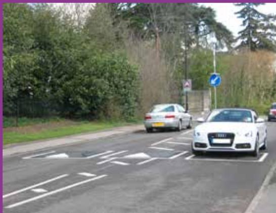
The precast units have to be laid on a 150mm bed of wet C40 concrete that must have at least 24 hours curing time before it can be opened to traffic. What with the reinstatement of the wearing course, the whole operation will take between 27-28 hours to complete one cushion.
