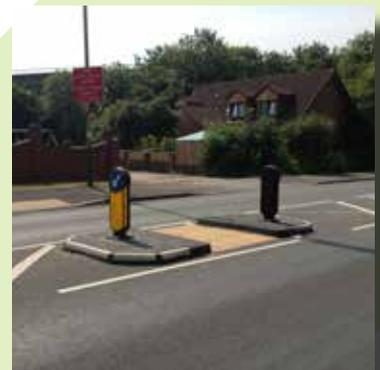
Rediweld products were used as construction alternatives in the form of islands and kerbing. The product due to the black and white markings also enhances the visibility of the kerb alignment along the route. The product also assisted in shortening the construction phase and additionally reduced the impact of the temporary traffic management at this traffic sensitive junction.
