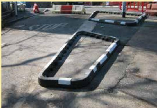
Site specific constraints were overcome by selection of this product which assisted engineers in achieving the required shape, final construction was then formed by infilling behind the kerb with asphalt. The pedestrian crossing construction utilised RediPave Refuge Islands and RediFix surface mounted tactile tiles.
