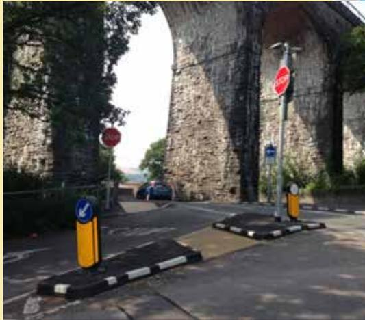
The RediKerb kerbing and RediPave Islands were installed by Rediweld within 3 days, with traditional materials this construction would have taken over 3 weeks. The scheme was the most cost effective solution causing minimal disruption, producing no spoil and requiring less traffic management.
